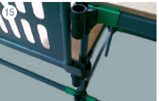
15 The bottom dasp of the deck bar should rest on the bottom handrail adapter. By eye this should leave a clear path through for the next handrail.
