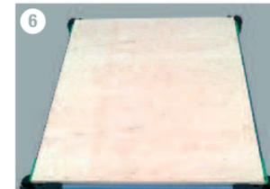
6 Complete the first unit by adding a deck panel, then continue to build by completing the frame using black and green rails.
